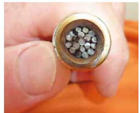
The break was clean and corrosion-free
